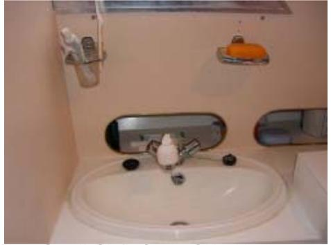
**New Small Sink;** fits in OK with the drain coupling to the shower outlet. The tap centre lifts out to form a shower head. This folds out of the way after use. I have utilised the original Seamaster fittings, just moved to a different position.
